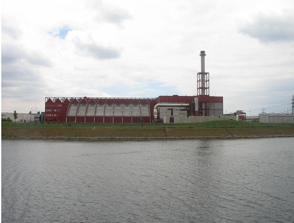
Fig 7. Thermoselect's Karlsruhe gasification facility (Germany)
